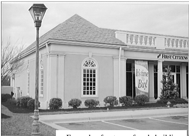
Example of a stucco façade building
