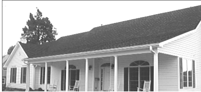
Example of Residential Style Building with Horizontal Vinyl Siding
