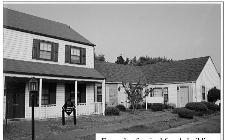
Example of a vinyl façade building
