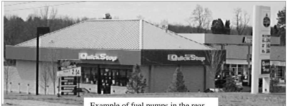
Example of fuel pumps in the rear
