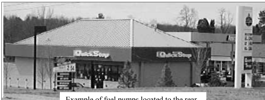
Example of fuel pumps located to the rear
