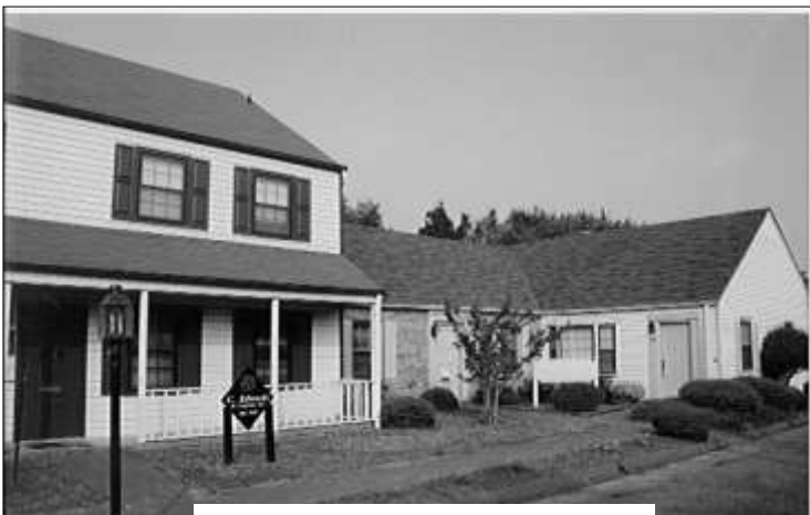
Example of a vinyl façade building
