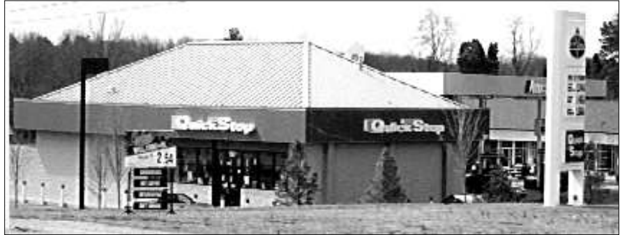
Example of fuel pumps placed to the rear of a building.
