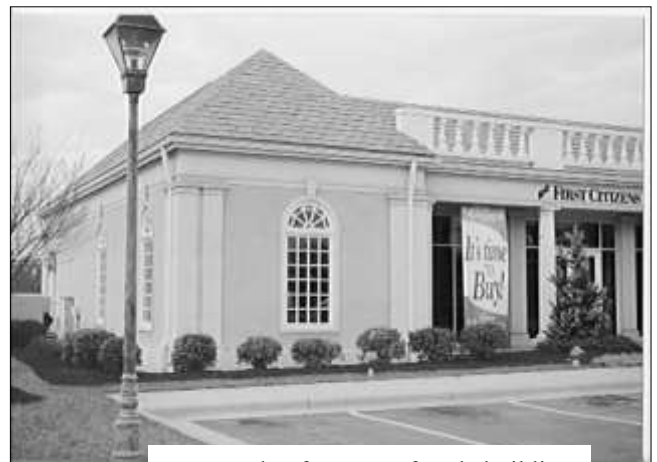
Example of a stucco façade building
