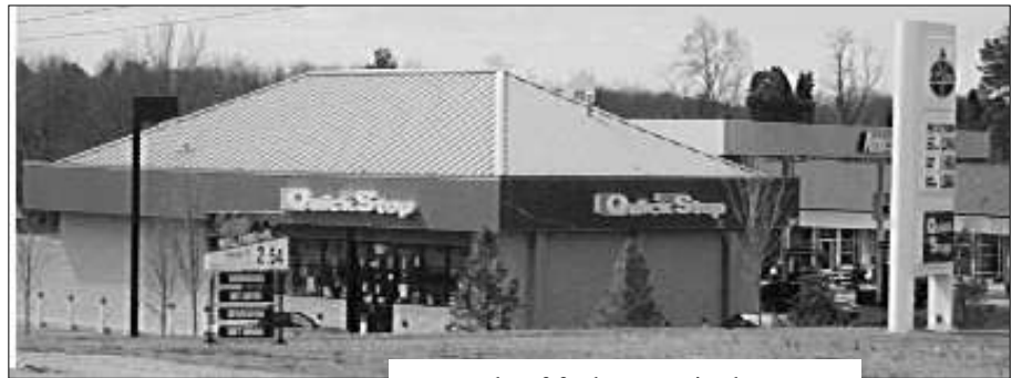
Example of fuel pumps in the rear
