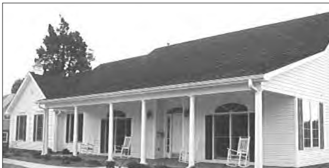
Example of Residential Style Building with Horizontal Vinyl Siding
