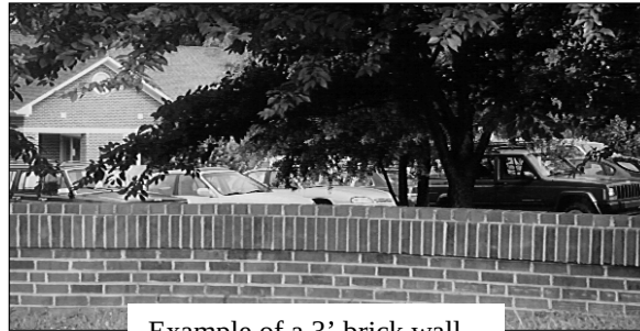
Example of a 3' brick wall
