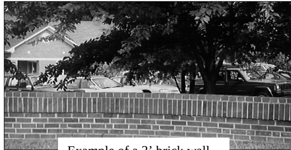
Example of a 3' brick wall
