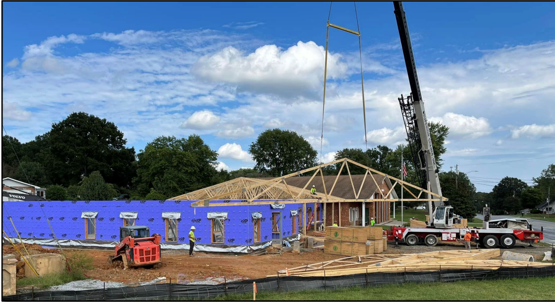
Photo: Construction at KFRD Engine 44 / BCFD Station 26
