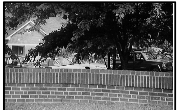
Example of 3' brick wall separating street from parking area
