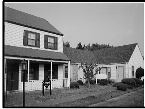
Example of a vinyl façade building
