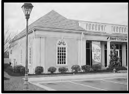
Example of a stucco façade building
