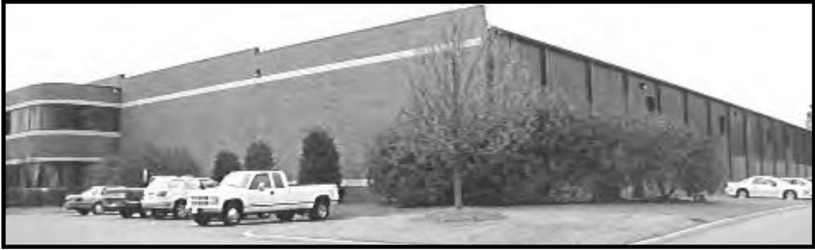
Example of an industrial building meeting the ICOD Building
