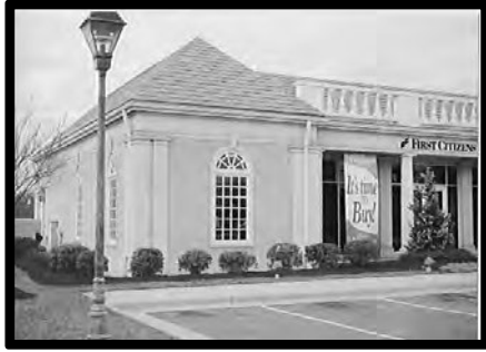
Example of a stucco façade building
