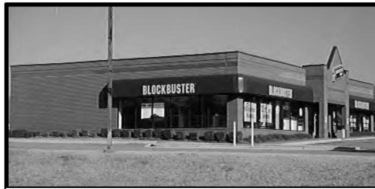
Example of a building meeting the HCOD Building Design and Material Standards
