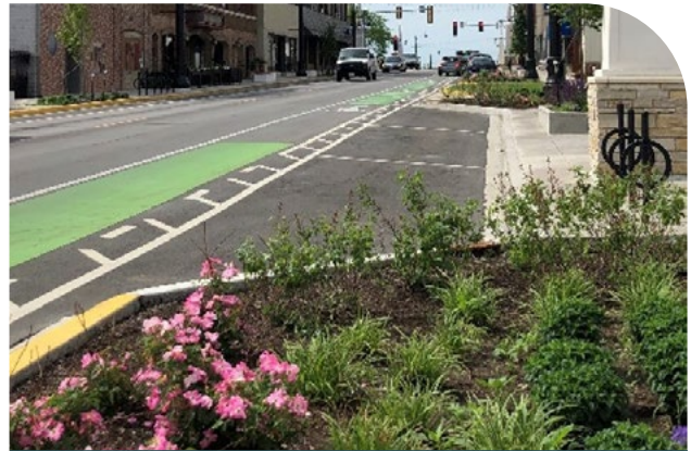
Rain gardens can fit seamlessly into other infrastructure improvements, like curb bumpouts.
