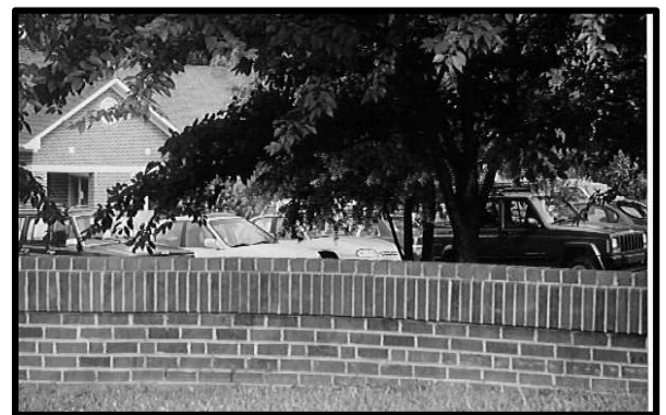
Example of 3' brick wall separating street from parking area
